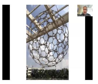
The next class, we are going to focus on something that looks like this. This is actually a geodesic dome that was built at IISER a few years ago, and this was part of a project, that was done here. And this is all assembled using, sticks, bamboo sticks and rubber bands and ties. And, and this kind of architecture, this geodesic dome always reminds me of the cytoskeleton because that is the kind of architecture.
