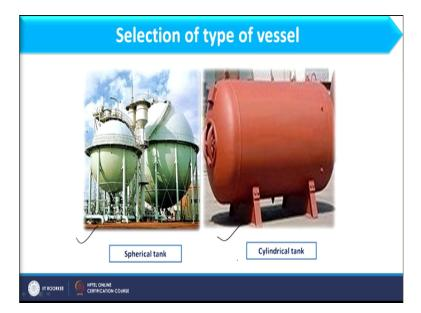
So here you see in these images I am having spherical tank as well as cylindrical tank, so it is looking like this. Now we need to discuss that what equipment we are going to design. Till now you have the idea that we are going to design the pressure vessel okay. And that pressure vessel should be related to chemical process. So what equipment we need to further design and would be the use of those equipment in the chemical industry again I am using the Onion diagram.
