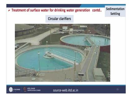
So, circular clarifiers are used in real life plants as shown in this figure. So, these are the clarifiers, we provide sufficient time to settle all the particles from this and from the top we collect the supernatant liquid for further treatment.
