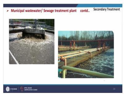
So, we can see here some picture. So, which shows the operations of the secondary treatment that is aeration unit. So, air is sent from the bottom and this type a big tank is used for the aeration purpose and for the biological degradation of the organic compound, it requires sufficient amount of aeration in tank.
