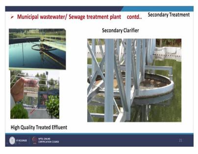
And then that is a aeration tank then it has to be settled. So, that we will be getting the sludge at the bottom and from the top we will get the clear water. So, these are the clarifier and here also clarifier, you see the water is seems to be very clear and this is high quality treated effluent as shown here. So, after secondary treatment, the turbidity of the water reduces significantly and it appears nicely as shown here becomes very clear.
