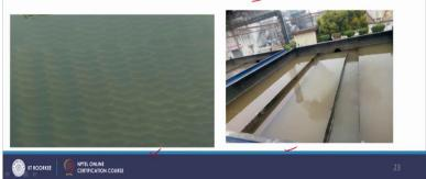
So, now, another important type of sedimentation unit which is used that is tube and plate settlers, these are some improved versions, the efficiency is more than the conventional sedimentation unit in this case. So, here this is our tube settlers and this is our parallel plates in our rectangular sedimentation unit. So, this installation of these plates reduces the requirement of height for the separation.
