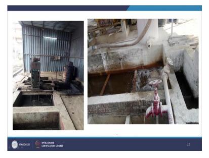
This shows the oil separation unit and this is the lime addition.
