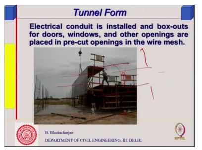
So this is whole thing is being lifted by a crane at the ground floor level so any openings you require you can always have pre-cut. And wires reinforcement is precast I mean pre-cut actually.
