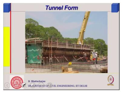
So they can, they can combine this is a fast construction actually and sustainable in the sense that you can make high strength concrete reduce down the materials and material cost, right.
