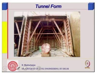
For example, this and this are fan you know heater and a fan, this is a turnbuckle, turnbuckle has took out, these are turnbuckle, so you rotate this you can see there is a rod sort of a thing this is actually handle. So, if you rotate this either it will close or it will open because there is a threaded portion inside here and there is a out you know thread inner inside thread and outside thread, there is a slip on which there is a thread and this is a rod on which there is a thread so you
