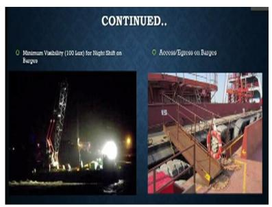
So, in this particular picture you can see this is the access and egress on barge. So, it has to be secured properly using structural steel material rescue teams shall be readily available at all the time to deal with emergency situations. Passenger vessel barges of under, 60 meters in length shall carry not less than 6 lifebuoys. Warning signs and notices shall be displayed all bollard ropes to be secured properly to avoid falling into the sea. So, what is the bollard ropes?
