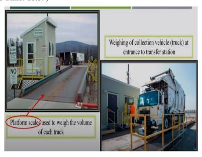
So I will show you some of the photographs in that way. This is the one particular weighing platform where the vehicle before entering the disposal site is getting weighed in this particular platform with the completely full vehicle and with this is like one photograph and also while coming back from the disposal site they empty weight also is getting measured.
