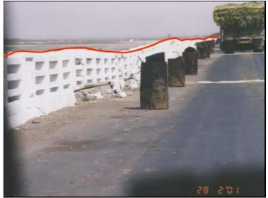
And this is the photograph of 2001 Bhuj earthquake in Kutch which is resulted in to the preservation of the S wave. So waved up surface if you take here, this is a bridge which shows a very beautiful preservation of the passage of the S wave here. This is on the bridge.
