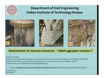
Now, here are examples of concrete structures where we could say that suspected alkaliaggregate reaction. And that is in this case the aggregates which we thought are largely inert are not really inert. And we have a reaction of aggregates with the sodium potassium and the hydroxyl ions in the cement paste and that is what is causing a deleterious action, including formation of cracks, appearance of the white gel, and so on.
