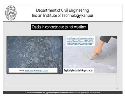
Here are pictures of cracks in concrete due to hot weather. Typical plastic shrinkage, cracks can be seen and we should also note that concrete may stiffen prematurely preventing proper compaction and proper finish or temperature of concrete may rise causing thermal cracking as it cools. So, this thermal cracking part we will visit once again when we try to study mass concrete but that is a slightly different variation of concrete conditions.
