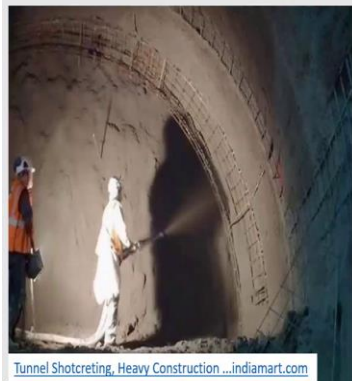
Tunnel Shotcreting, Heavy Construction ...indiamart.com
