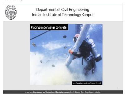
And this picture brings it out even more clearly for the diver is holding a concrete pipe and placing the concrete. So, we can see that the amount of wash out as far as cement is concerned is much less than you would expect and we can still see a lot of fish in the region.
