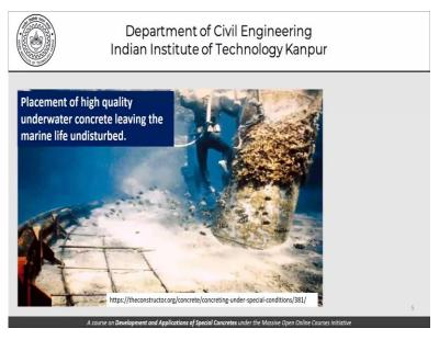
Moving forward this is another picture where concrete is almost being placed and we can see that placement of high-quality underwater concrete leaves the marine life largely undisturbed and you can see fish freely moving around this construction site. And you can see a diver trying to do certain operations.
