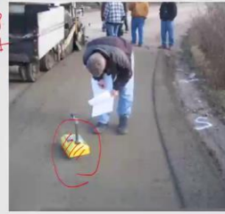
Measuring density of RCC using Gamma Densitometer
