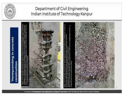
We have seen this picture before and we know that this honeycombing is a result of the inability of the concrete to flow around the reinforcement and that is the whole backdrop in which we are talking about self-compacting concrete. This is a similar picture for honeycombing and we have seen this before.
