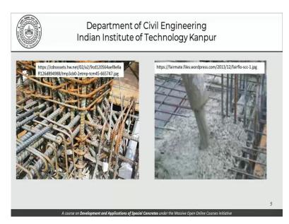
Now moving forward this is a real picture of a RC member and we can see that there is a huge amount of congested reinforcement. And concrete is expected to flow around this reinforcement and that is what has given rise to the need for the self-compacting concrete. That is impossible virtually to have a needle vibrator trying to get into the reinforcement that is shown here and try to compact the concrete.
