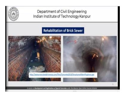
This picture here is rehabilitation of a brick sewer lining. So, you can see the deteriorated brick sewer here, rehabilitated into a sewer line which is something like this. Again, loss of cross section, yes, but a renewed sewer line, rehabilitated sewer line.
