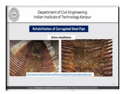
Now let me show you some examples of shotcreting being used for rehabilitation works in particular before we close our discussion for today. This is the rehabilitation of a corrugated steel pipe, so you can see that there is heavy corrosion as far as the steel pipe is concerned.
