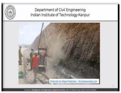
Moving forward, this shows the application of shotcrete in the case of slope protection, which is something very important when we are working with hilly areas where we are trying to stabilize the slopes. And trying to create infrastructure such as roads, canal lining sometimes we use this though that necessarily does not have to come under the slope protection banner. But yes, the application or the condition of application is more or less what is shown somewhere here.
