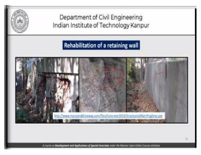
This is rehabilitation for retaining wall; again, we can see the rehabilitation including some kind of a mesh being placed first in position and then the concrete being deposited to strengthen the retaining wall which was possibly deteriorated to begin with.
