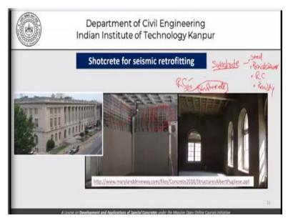
This picture here is for shotcreting operations for seismic retrofitting. And you can see reinforcement panels in the walls and we have a renewed structure which is more compliant with the different standards that we may have for seismic performance of structures compared to those standards that were prevailing when the original structure was built. So, one advantage of using shotcrete in the repair works especially is that it works with any of the substrate materials.
