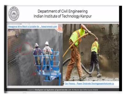
Moving forward this picture here particularly shows a more complicated form of deposition of shotcrete where the people here the operators, the nozzleman they are being lifted to a position, so that they can reach the place where the shotcrete is being deposited. And you can imagine that these 2 here is you should be able to see that we are trying to do reinforced concrete here. That is there is a certain amount of reinforcement involved.
