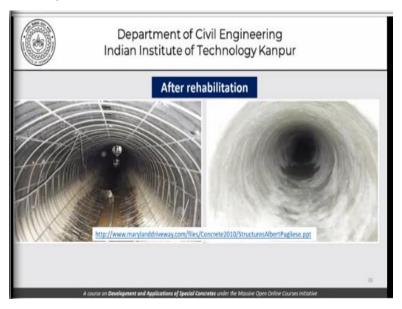
And this picture here shows the pipe after rehabilitation using shotcretes. So, what has happened of course is that the corrugated steel pipe has now got a lining of the concrete inside. We have lost some diameter but we have saved or we have recreated the pipe in a different form.
