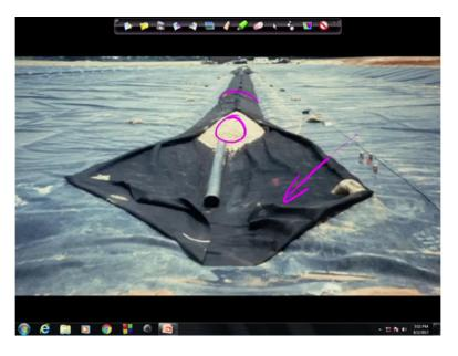
So this is also called like a fish bone design for leachate collection. So that is the head and the middle pipe that you saw and this is your geotech style that I was talking about. So this is your geotech style part that is the black part that you see is the geotech style and then this is the pipe the pipe has perforations where the waste is getting collected sorry the leachate is getting collected.
