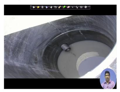
So that is how the leachate will be and then we will put pump in these wells because these wells will be accessible during the landfill operation. So this is another picture of those like a wells and then you can see the picture from inside you see the pipes coming in right now it is
