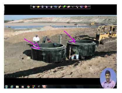
So this is some pictures of those leachate wells which you saw in this case earlier. So as you can see there is a landfill on the other side of this burmp we have a this liner system leachate collection system and then the leachate collection system where pipe will come into these and the leak detection system pipe will come into these particular well.
