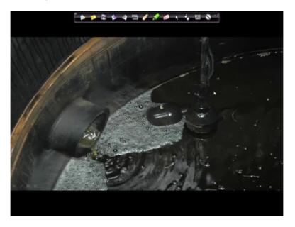
And this is how the leachate looks like you can see this nasty colour leachate which is coming out from this from this landfill. So you see those here based on the level of the leachate in this tank. The pumps kick in and the pump will pump out this leachate to the leachate treatment system. So it will be piped to the next treatment unit.
