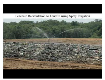
As you can see over here the leachate is being spread around this system where this it is being used the spray irrigation for the for this to recirculate the leachate.
