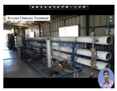
RO is used quite extensively these days especially if you want to make water to be really clean and that can be reused as portable water. So you can have a RO system is used for that.
