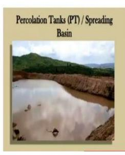
Now next is the Basin and percolation tanks so this is the most common method of artificial recharge in this method water is impounded in the series of basin of percolation tanks. So, this is a series of you can see here some small basin is there and this basin the water is stored so this method is the most common method of artificial recharge here water is just stored in the basins or percolation tank.
