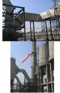
85 m tall, discharges flue gases from 2 boilers (43 MW power plant)
