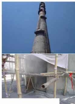
Heavy ash deposition at bottom Pungent smell of sulphur bearing gases
