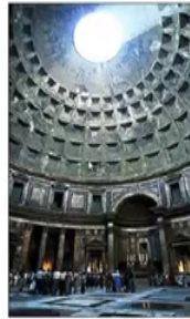
Pantheon dome, Italy Completed in 123 AD 142 ft. diameter; weight reduced by waffle-like depressions Opening at top: 'Oculus'
