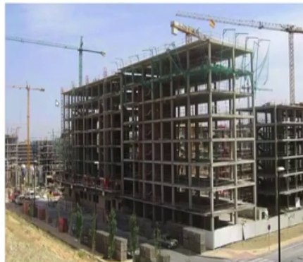
Grid of columns and beams (cast integrally with slab); walls infilled later
