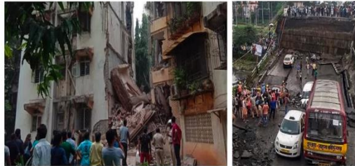
Building/bridge collapses due to known/unrestricted corrosion and poor maintenance/repair
