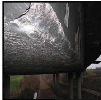
Figure 2.26 Fire spalling from a fire under a bridge. The heat source was solvents burning under the bridge coming from a lorry on the bridge. Photo Lars Boström.
