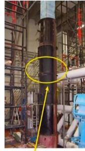
Column prepared for high strength concrete pour
