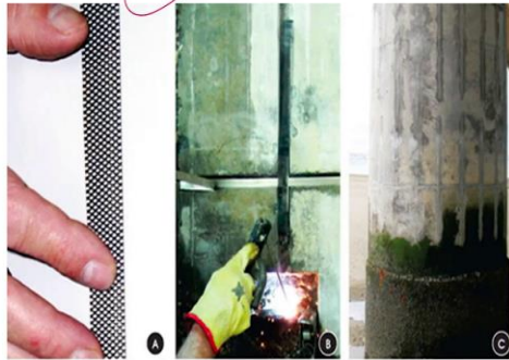
Activated titanium ribbon anodes
