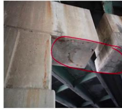
Cracking at the underside of bent-caps due to corrosion
