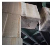
Cracking at the underside of bent-caps due to corrosion
