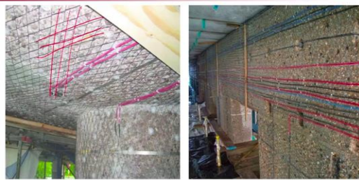
Activated titanium mesh is fastened to the substrate concrete surface and ready for overlay
