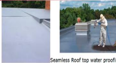
Seamless Roof top water proofing
