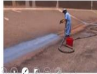
Crack filling and water proofing of Canals, Dams
