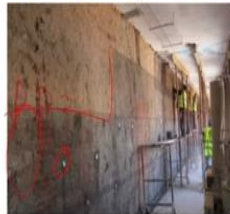
Steel mesh application on the site (interior leafs)
