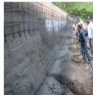
Application of shotcrete
