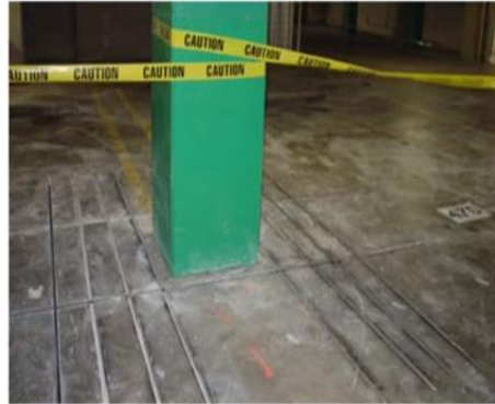
Surface grooves cut for NSM CFRP rods for negative moment bending upgrade
