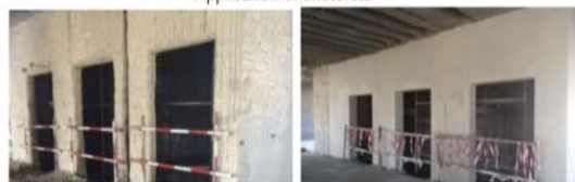
Elevator walls before (left) and after (right) the repairing works
