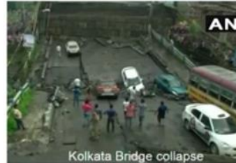
Kolkata Bridge collapse
