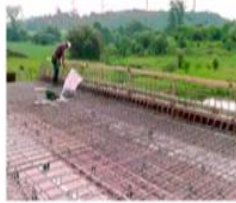
Stainless steel rebar on a bridge deck of the 407 Highway, Toronto.
