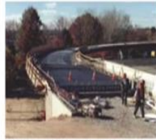
165 tons of 2205 (duplex) stainless rebar were supplied for the new ramp of the Garden State Parkway in New Jersey (1998)
