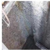
Inside view of a concrete manhole
