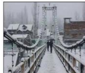
Snow-covered foot bridge
