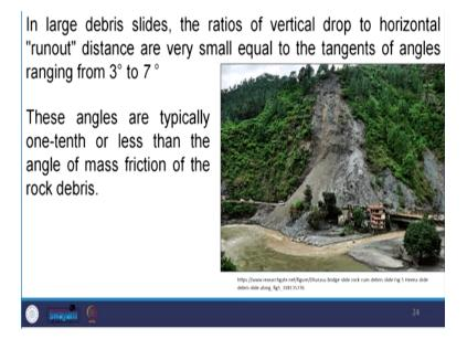
In large debris slide, the ratio of vertical drop to horizontal run out distance is very small equal to tangents of angle ranging from 3 to 7 degree; these angles are typically, one tenth or less than the angle of mass friction of the rock debris. So, if you remember our earlier class, when we started about this mass wasting, we are talking something about the strength, this angle of repose or so. So, here the large debris slide, the ratio of vertical drop to horizontal or not.
