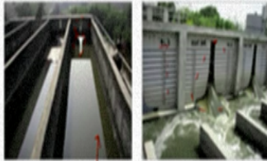
Figure 5.31 Typical installation of proportional flow weir
