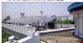
60 kWp installed on rooftop in Ballarpur Area Office, Western Coalfields Limited (WCL), Maharashtra
