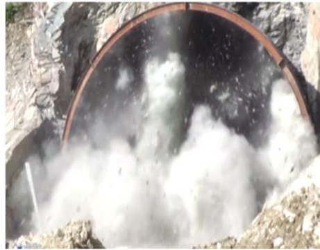
First blast at south portal of tunnel
