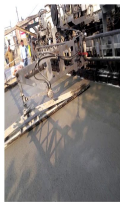
Surface finishing in progress
