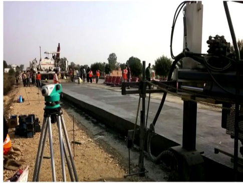
PQC after Construction
