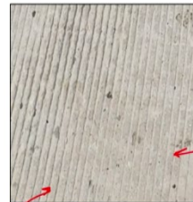
B- Texturing done in Plastic Stage
