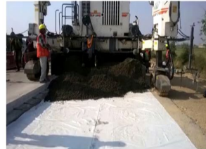
Starting of PQC Laying Work
