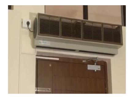
Why we are showing you this is that at the entrance of the lab, you can see an equipment placed on top there is an air curtain again. So, the air curtain will allow to push dust particles outside. Now, Seetharam will enter the lab as he enters the lab you can see that the air curtain is falling, that air curtain will ensure that the dust particles do not enter inside.
