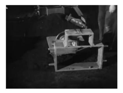
Here, we see a hand molder putting down the bottom half of the pattern onto the wooden board that will form a temporary support.
