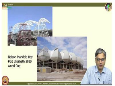
another picture of a truss which is a space truss you have this occupying in three dimensions.
