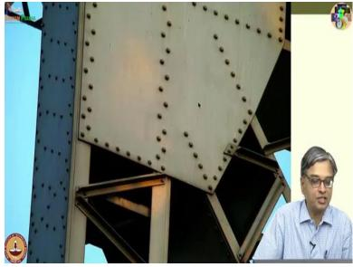
you that these are rivets that is how the joints are made.
