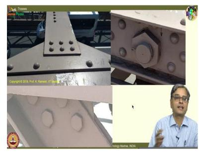
could also see some segments they have a bolted connection. In another section they have a completely connected with bolts.
