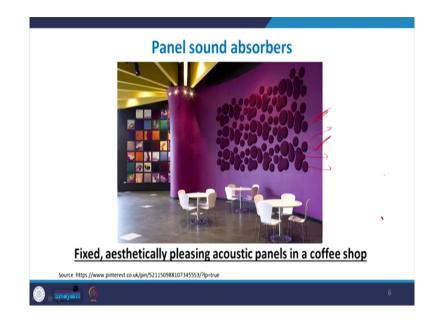
So, here in a coffee area. You have lots of these boards. So, to a viewer it may seem like this is sort of a decoration wall decoration or sort of done for aesthetic purpose, but the main reason for using these panels is to reduce the noise. So, these are actually acoustic panels which two of you and may look like aesthetic elements.
