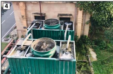
Cooling Tower and the outdoor unit of centralized HVAC system (anonymous location, Haridwar district, Uttarakhand)
