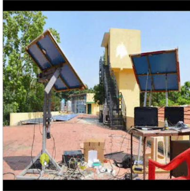
Ashith – Solar Energy
