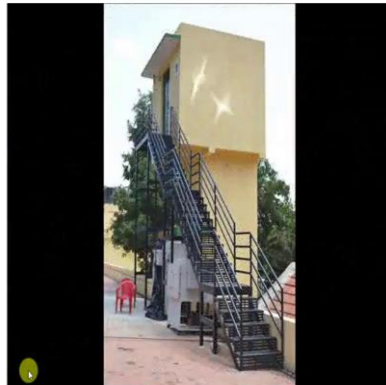
Ashith – Solar Energy
