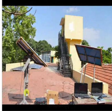
Ashith – Solar Energy
