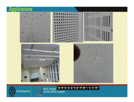
And these are these are for particular purposes. So, these are all commercially available knowing the reverberation time of the room; required in the room such kind of area calculations and such kind of installations, such kind of acoustical absorber has been installed in such spaces.
