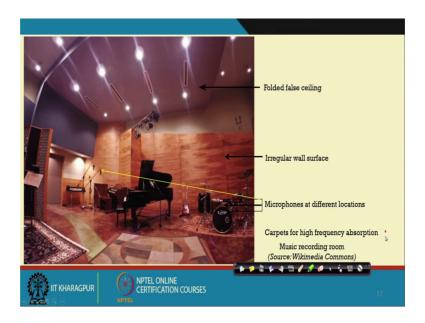
Here is another picture taken from the Wikimedia Commons. Here you see the irregular walls surface, irregular folded ceiling, and carpets on the floor different instruments located and the number of microphones which are all following the rule of three.
