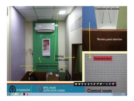
So, this is another view from the on the recording area. So, what you see on the walls? Let us see what is there in the walls you see there are absorbing surface all around starting from the ceiling and all the walls. So, these are primarily required for these particular kind of spaces here you see the slanting double glass, here this has been located in this fashion.
