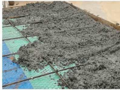
Pre cast ferro-cement roofing (under construction)
