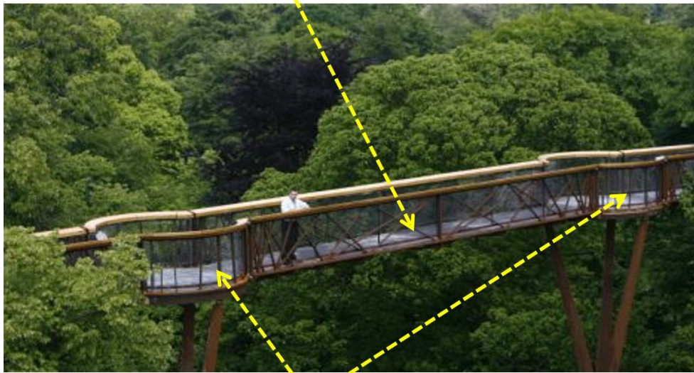
Vertical Web like member near the Support
