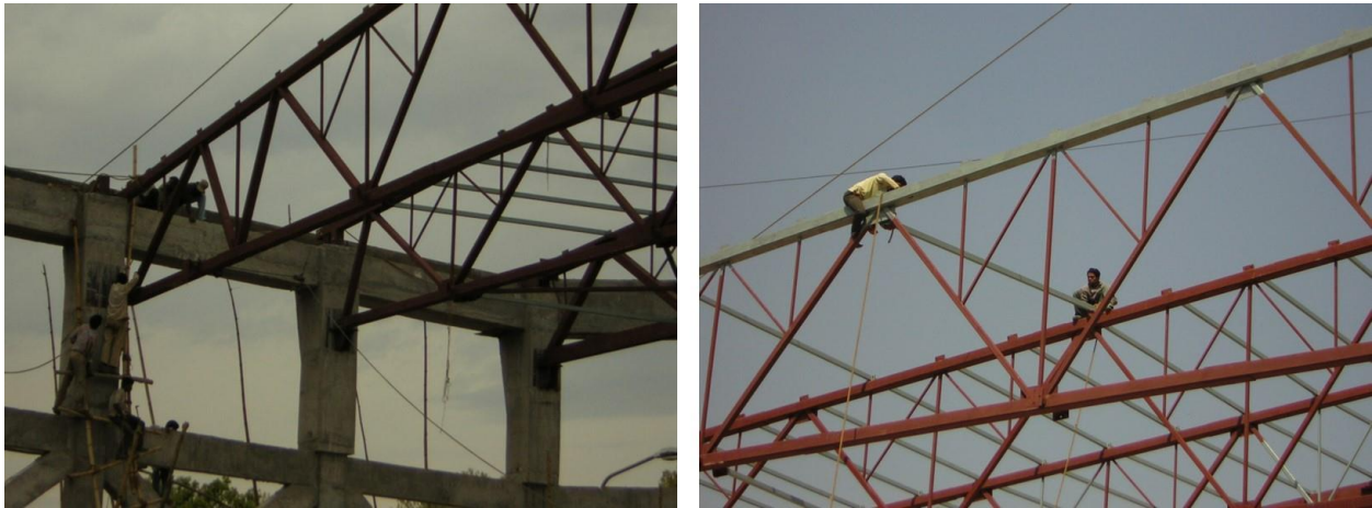
Figure 18 : the erected Truss
