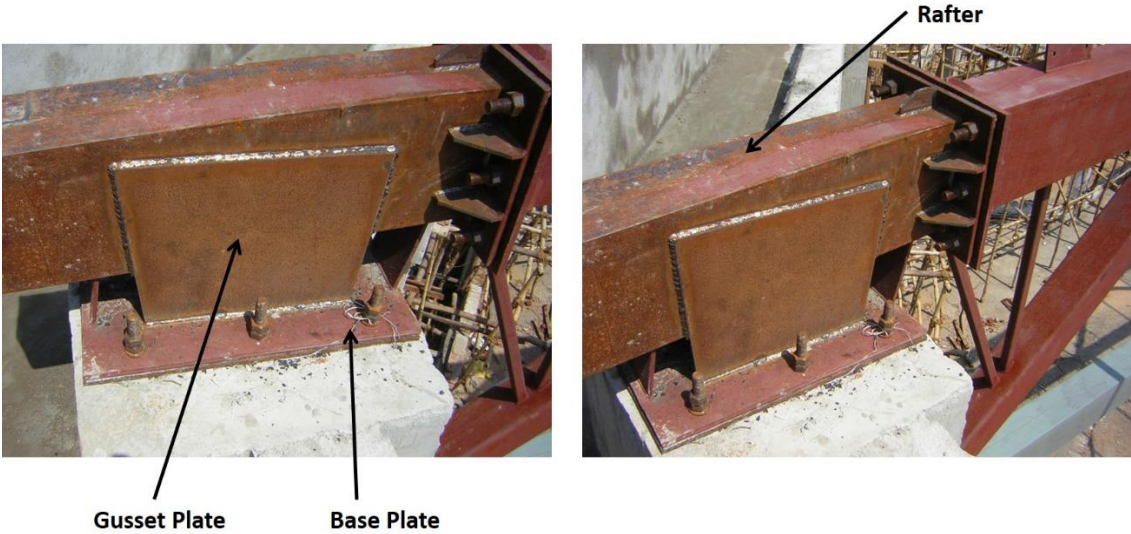
Figure 17 : gusset plate, base plate and rafter
