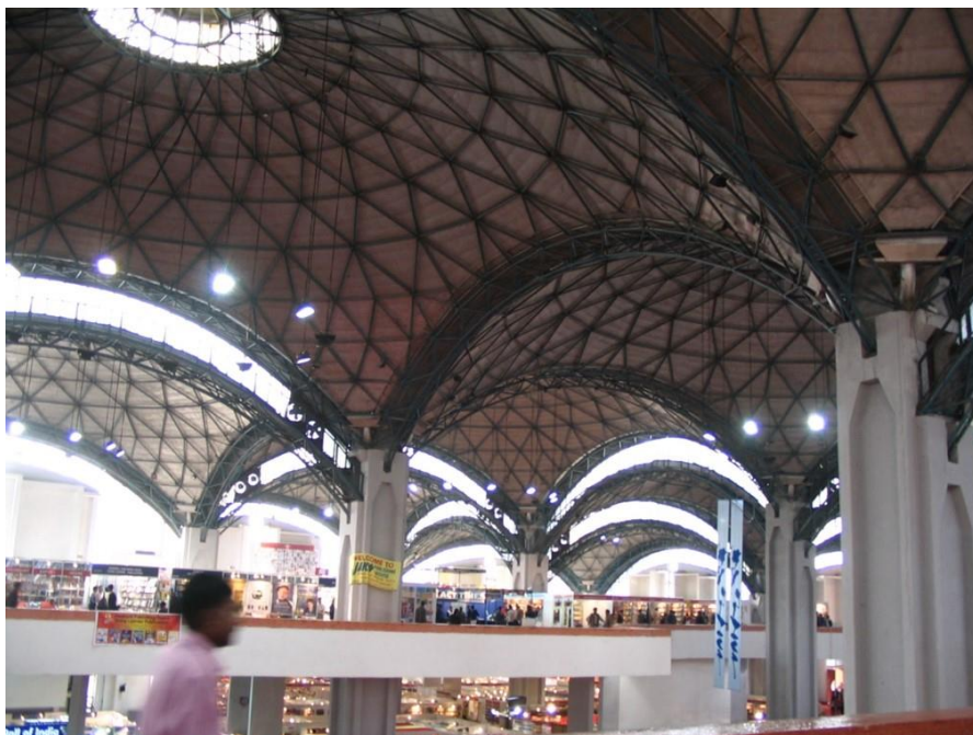
Figure 25 : dome shaped Space-Frame structure, Hall No. 18, Pragati Maidan, New Delhi
