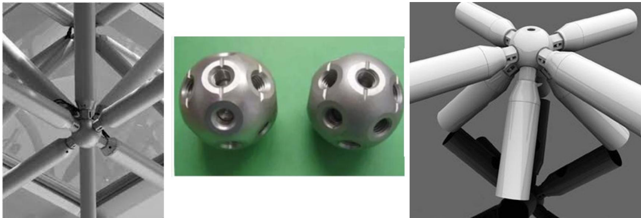
Figure 13 : threaded connection
