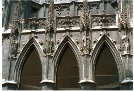
Figure 6 Gothic Arch (pointed)
