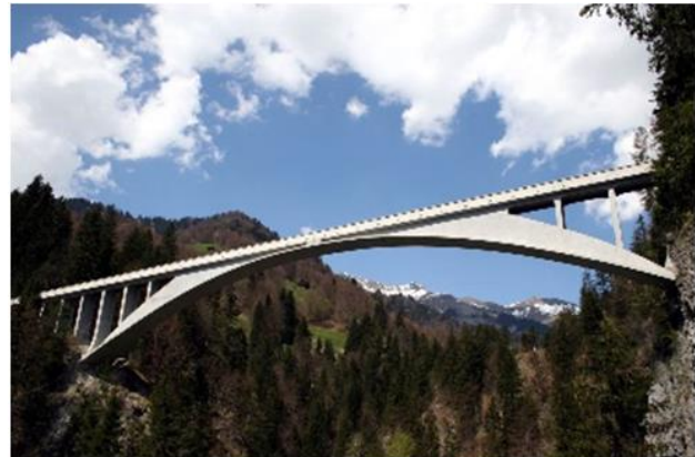
Figure 14 The Salginatobel Bridge, Schiers, Switzerland
