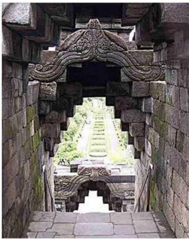
Stone corbelled arches at Borobudur, Java, Indonesia
